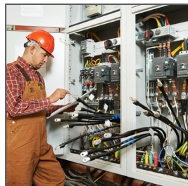
Industrial Electrical Box
